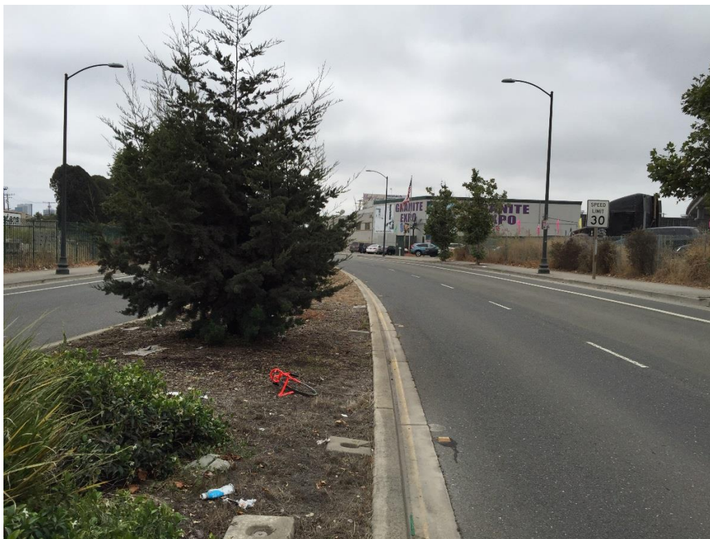
Photo 2: Southbound Mandela Parkway, looking south
