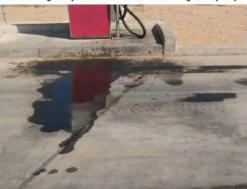
Allow sheet runoff to flow into biofilters (vegetated strip and swale) and/or infiltration devices. Utilize sand filters or oleophilic collectors for oily waste in low concentrations. Clean out oil/water/sand separators regularly, especially after heavy storms.
