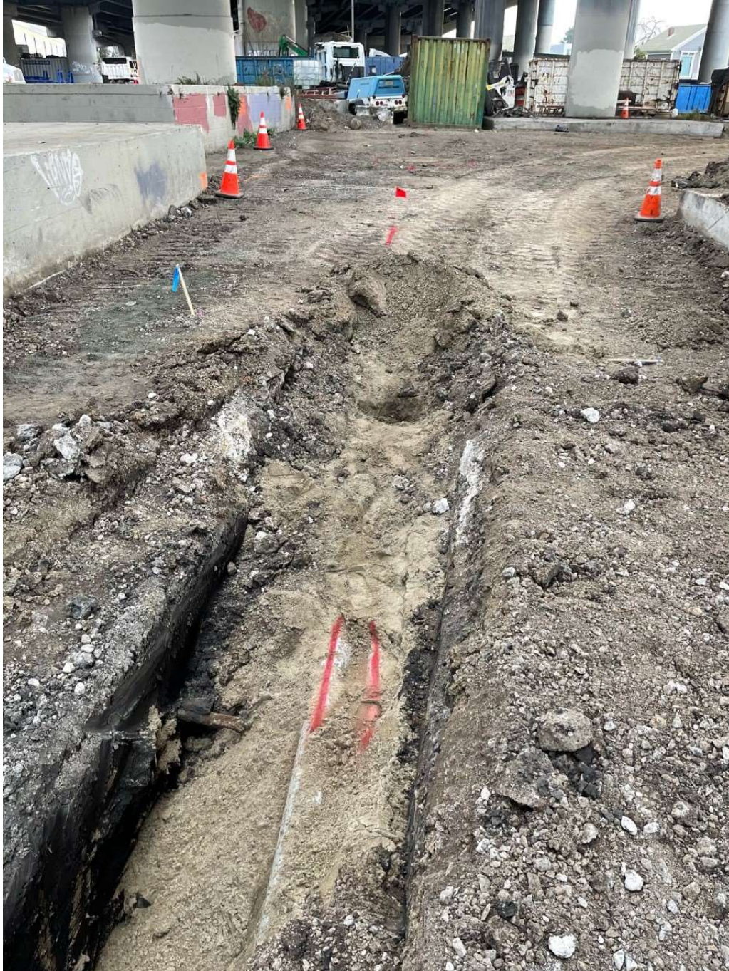
PG&E LINES IN CONFLICT WITH BIORETENTION AREA 1
