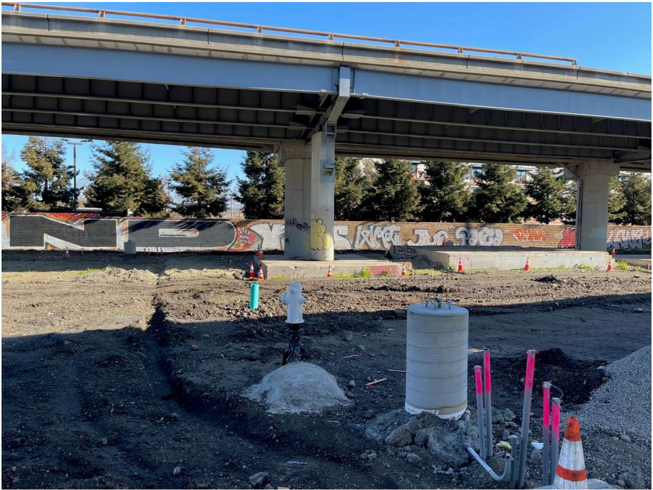
FIRE LINE COMPLETE – LIGHTPOLE FOUNDATIONS COMPLETE
