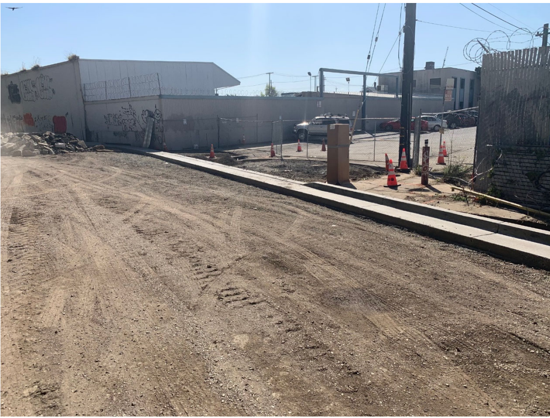
ETTIE STREET GATE REMOVED, CURB POURED, NEW PG&E PEDESTAL
