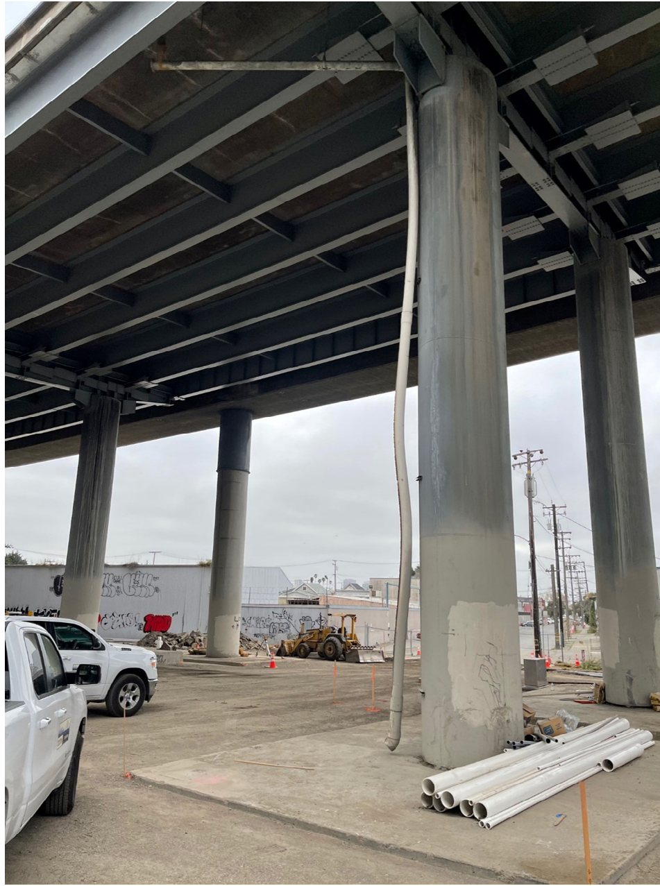
CALTRANS EMAILED ABOUT DISCONNECTED FREEWAY DRAINS – SITE HAZARD
