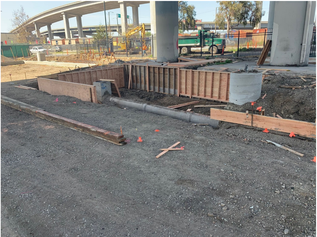
BIORETENTION AREA ALONG MANDELA PARKWAY – BEING FORMED FOR POUR THIS WEEK
