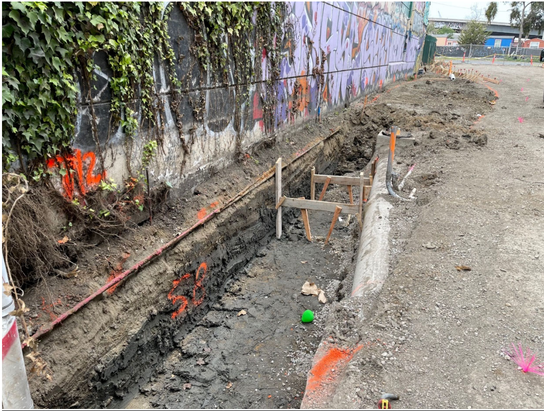
BIORETENTION AREA ON SOUTH PROPERTY LINE – UTILITY CONFLICTS RESOLVED
